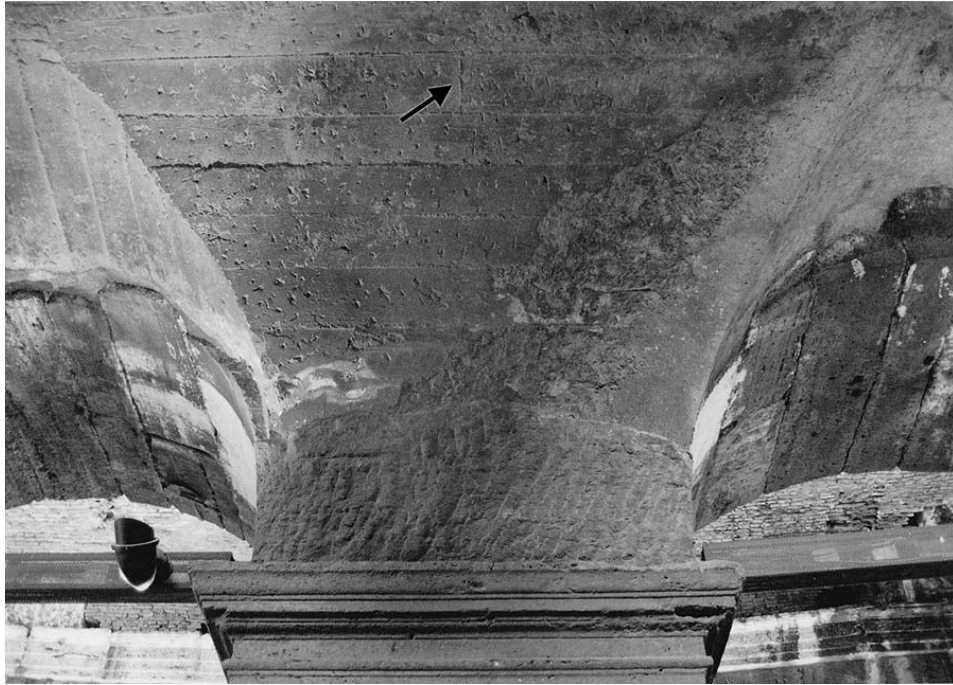
FIGURE 10. Groin Vault in the AMPHITHEATRUM FLAVIUM , 80 CE. Note the horizontal lines indicating original formwork. These lines are the often the only method for reconstructing formwork and centering, as there is no archaeological record of how they were actually employed (Lancaster 2005, p. 38).
