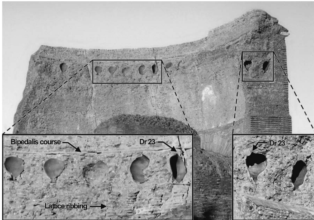
FIGURE 15. Exposed amphorae, as used at the Mausoleum of Helena, southeast Rome, ca. 330 CE (Lancaster 2005, p. 69).
