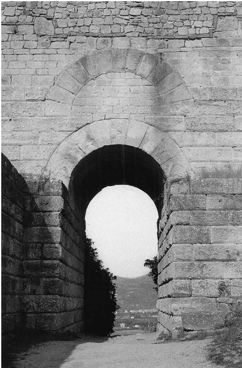
FIGURE 13. Ribbed vaulting, PORTA ROSA gate, Velia , third century CE (Lancaster 2005, p. 87).
